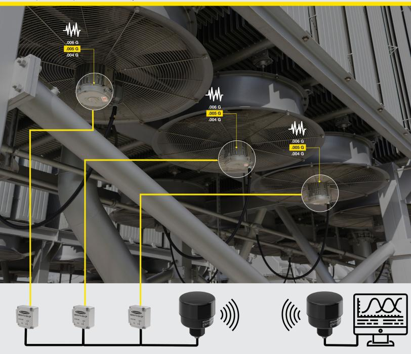
Ramping up to Industry 4.0 has never been easier. Speed-up and simplify installation by wirelessly communicating to any Modbus device using R70 Serial Data Radios. Information is effortlessly communicated over the air via a wireless communications network and terminated at the machine or an industrial controller. Monitor critical assets in a SNAP.
