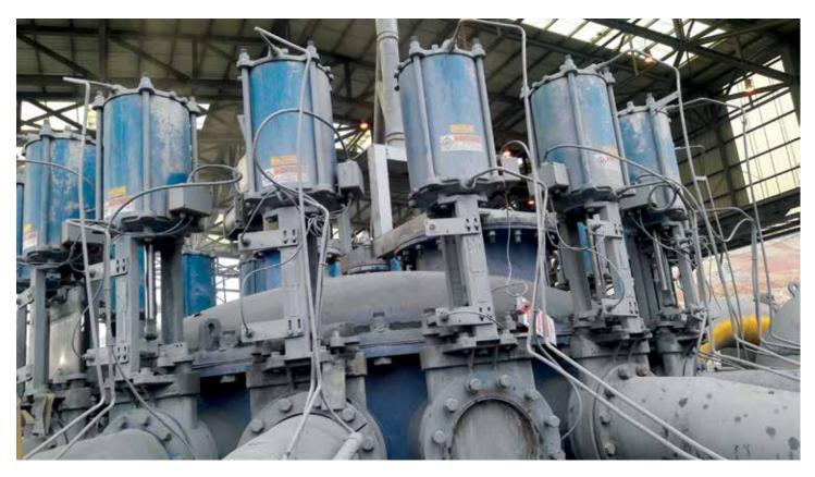
Ten 10" (250mm) DeZURIK KUL Urethane Lined Knife Gate Valves are installed in a hydrocyclone nest at a copper mine. These valves lasted two times longer than the competitor's valves in this service.
